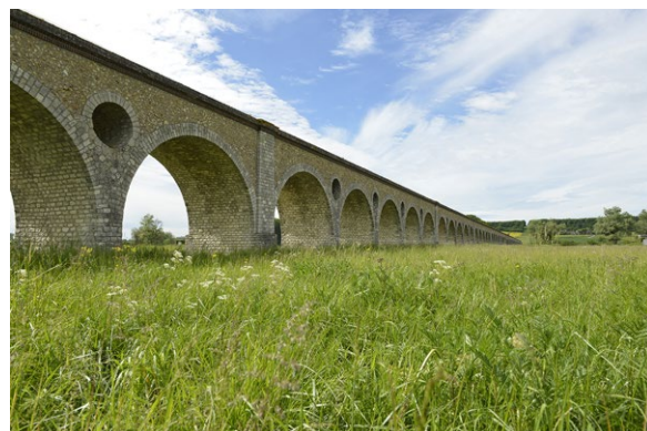
Avre aqueduct (Eure-et-Loir)
