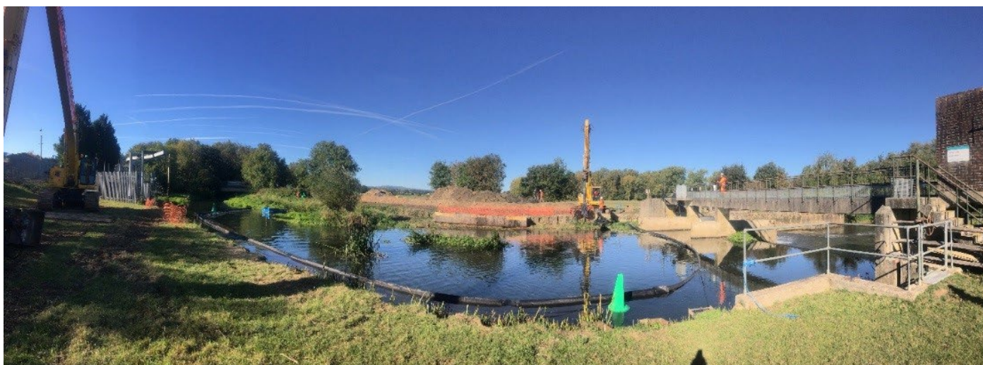
Fig.3 - Western Rother desilting upstream of Hardham weir, October 2018
